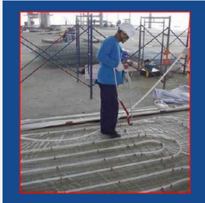
Hydronic Radiant Cooling System
